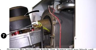
Remove the inspection hatch, fan, burner and gas block unit.
